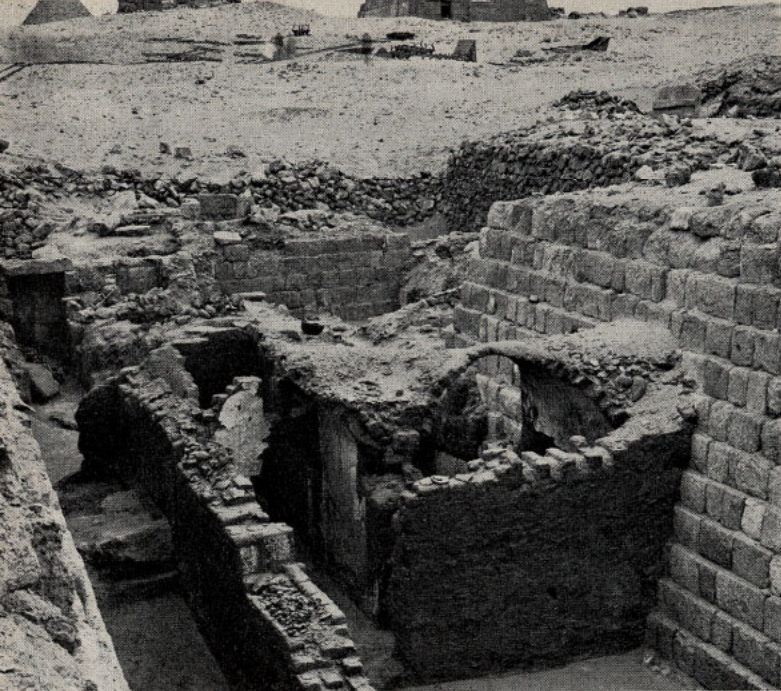
6. Brick chapel of Kanofer (G 1203) situated in the street behind Wepemnofret's tomb. Remains of two barrel vaults are visible.
